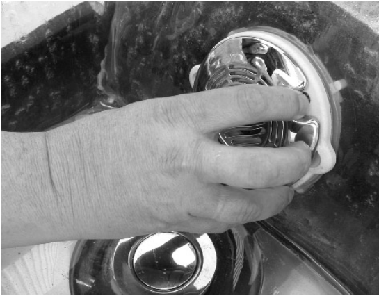
Remove screen by turning counter-clockwise.
